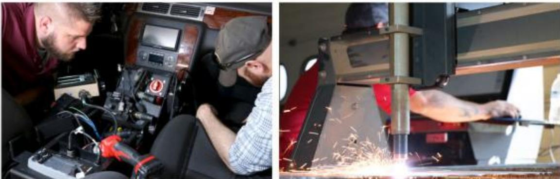
LEFT: Integrators perform testing to ensure all electrical and radio components inside an integrated center console are performing correctly. RIGHT: An automated plasma table is cutting out custom mounting brackets to securely
